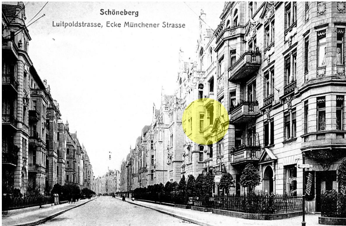
Luitpoldstrasse 27, Berlin-Schöneberg. It was the second time he rented rooms on Luitpoldstrasse. In WWII the whole street was erased; there is not one of the old houses left.
