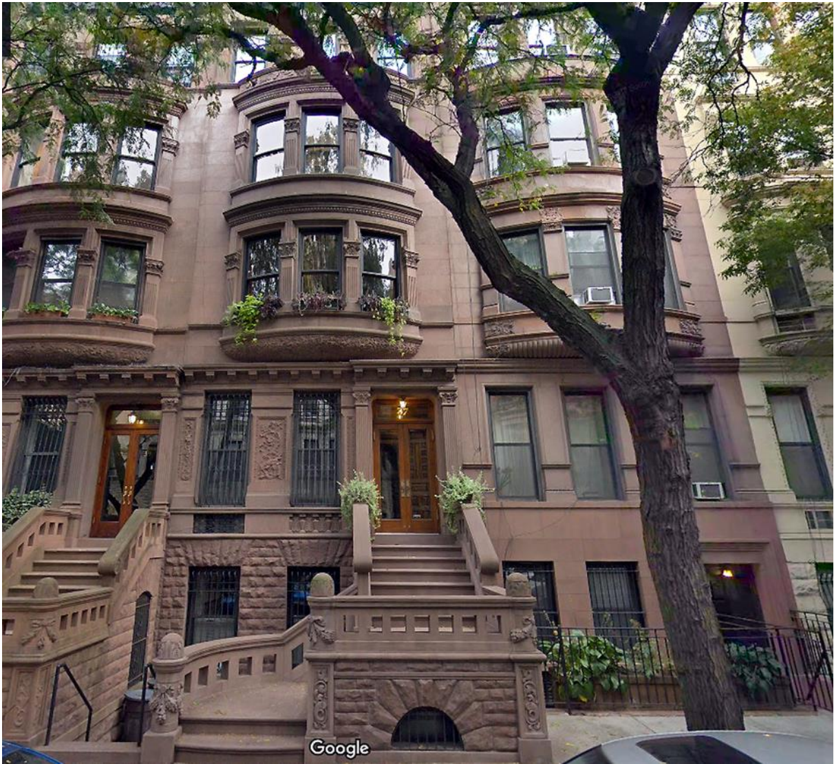
35 West 87th Street, New York City. The building has been thoroughly revamped c. 2015.
